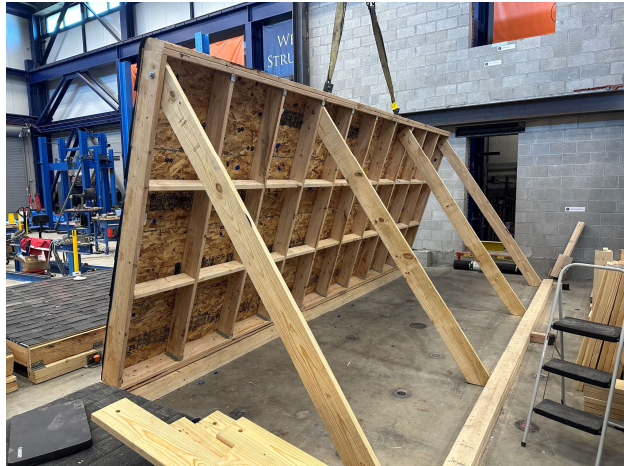
Figure 2. Vertical orientation of frame allows for documentation of nail holes on underside of sheathing.
