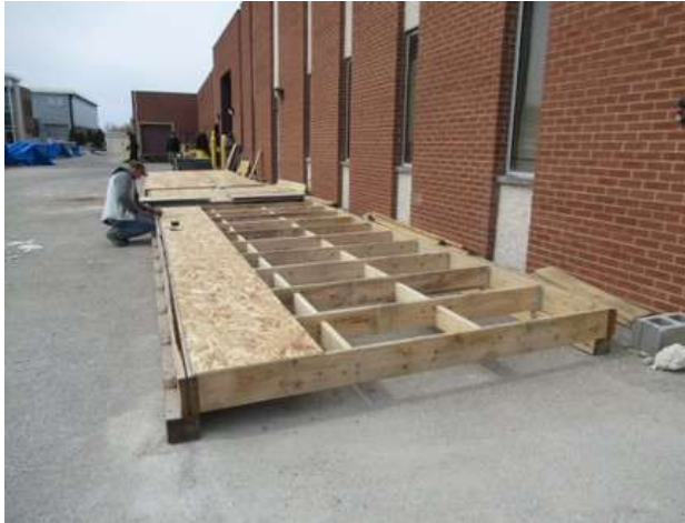
Figure 6. Sheathing installation with frames in a flat position.
