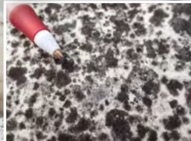
Photo 2 Biological growth (mildew) on the surface of Single-ply membranes in hot humid southern climates, markedly decreases solar reflectivity.
