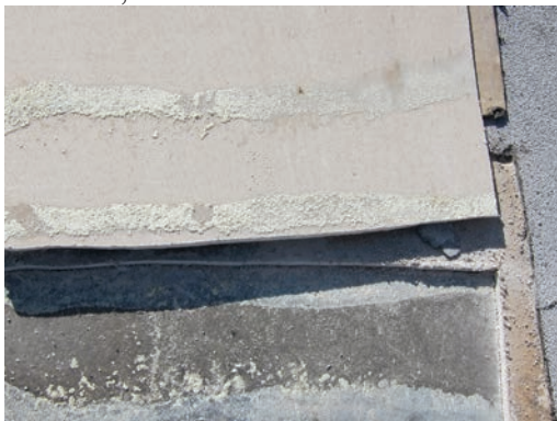
Fig.4 Soft, off ratio foam adhesive coming apart; cohesive failure within the foam
